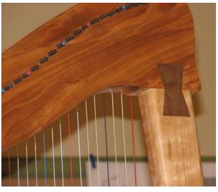
Joinery detail. The duthman is structural.
